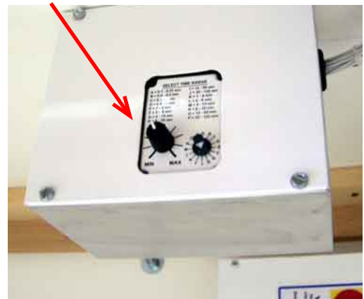
Relay timer adjustment
